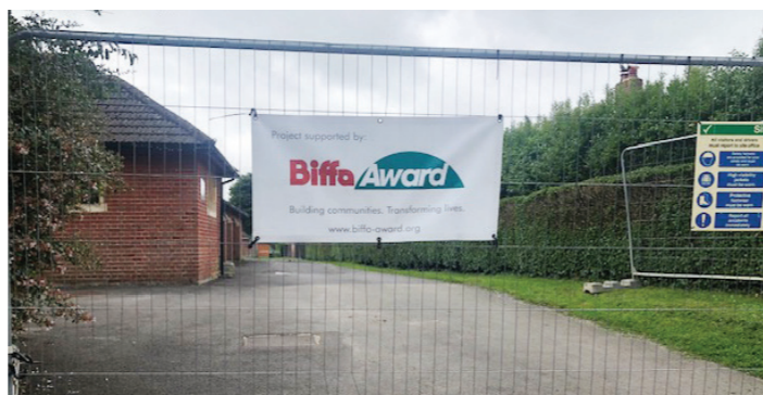
Renovation work has been extensive
