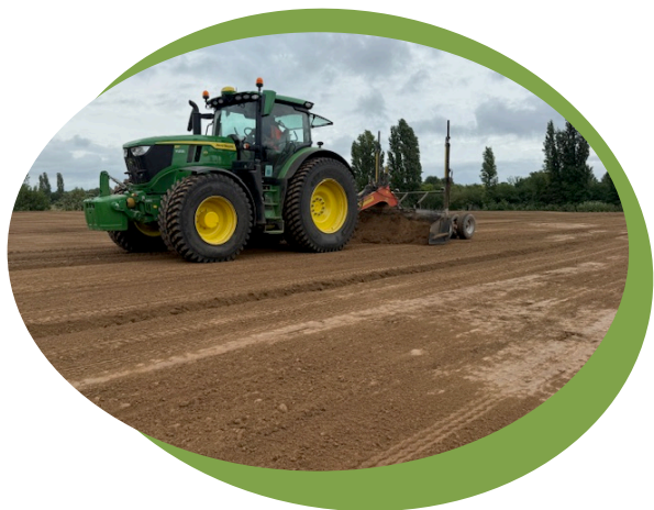
Grader levelling the ground
